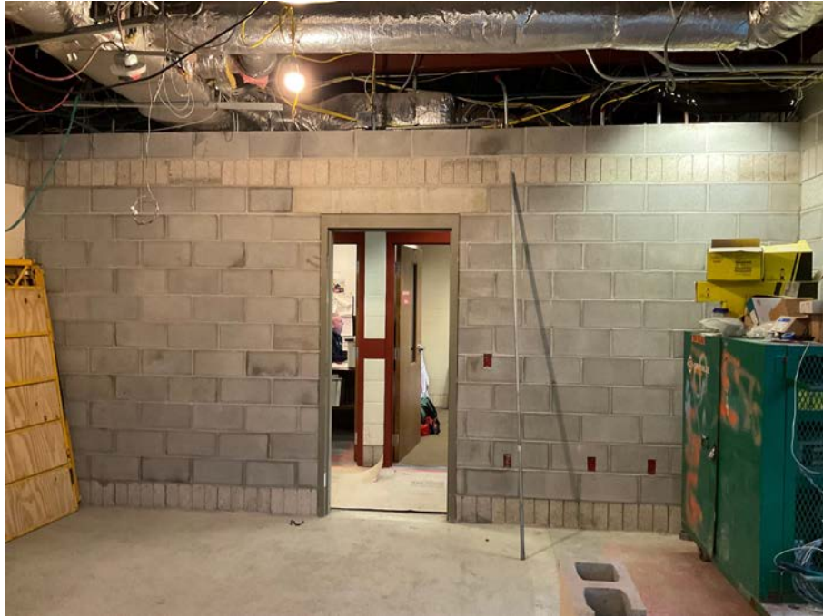
Old Dispatch Looking North
