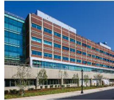
Gant Building Renovation Phase I-II
