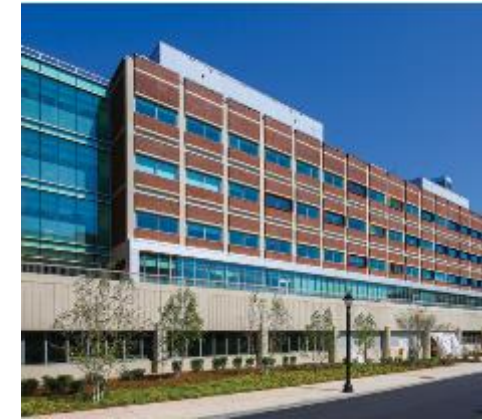
Gant Building Renovation Phase I-II
