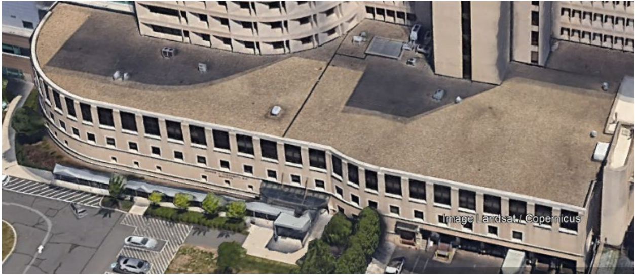
BUILDING F (CANZONETTI BUILDING) ROOF
