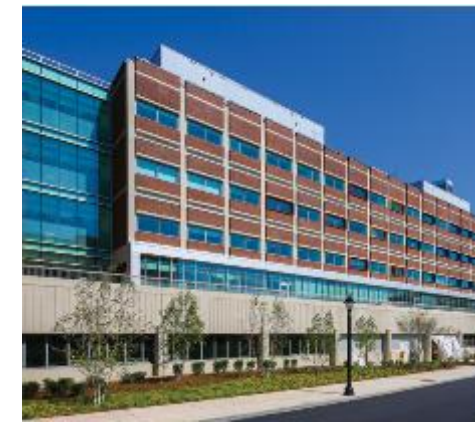
Gant Building Renovation Phase I-III
